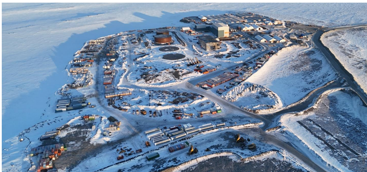
Goose Project site laydown area – April 2024
