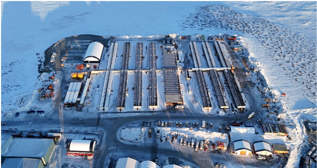
Goose Project accommodation complex overview – April 2024
